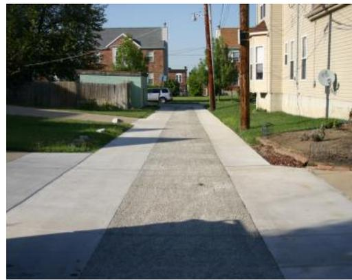
**Cardinal Alley (Left):** This old brick alley was converted into a pervious asphalt alley. **Eads Alley (right):** This former asphalt alley was converted into a porous concrete alley. Photos courtesy of CH2M HILL, Inc.
