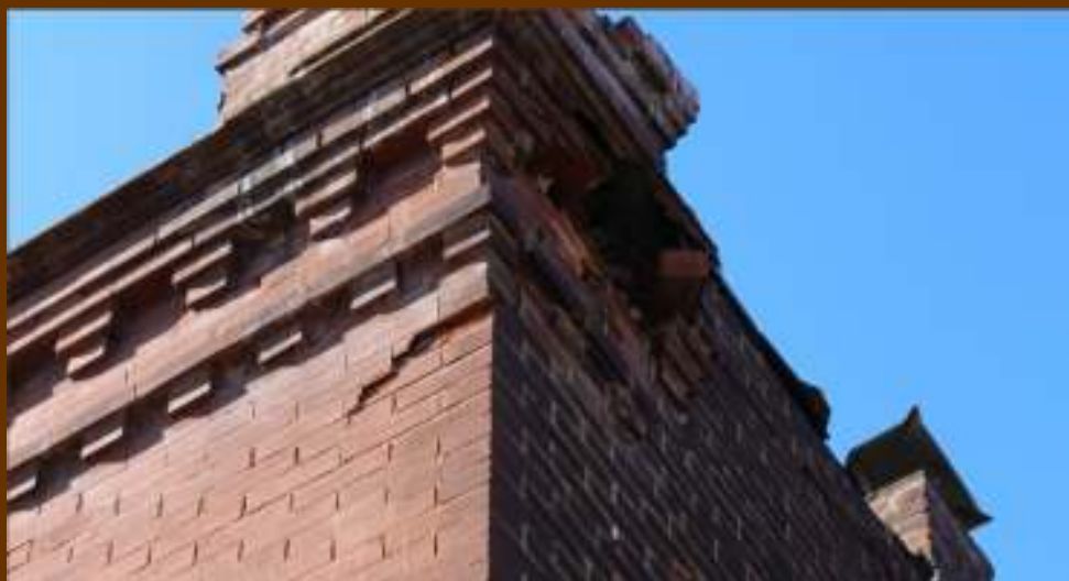
PARAPET DAMAGE
