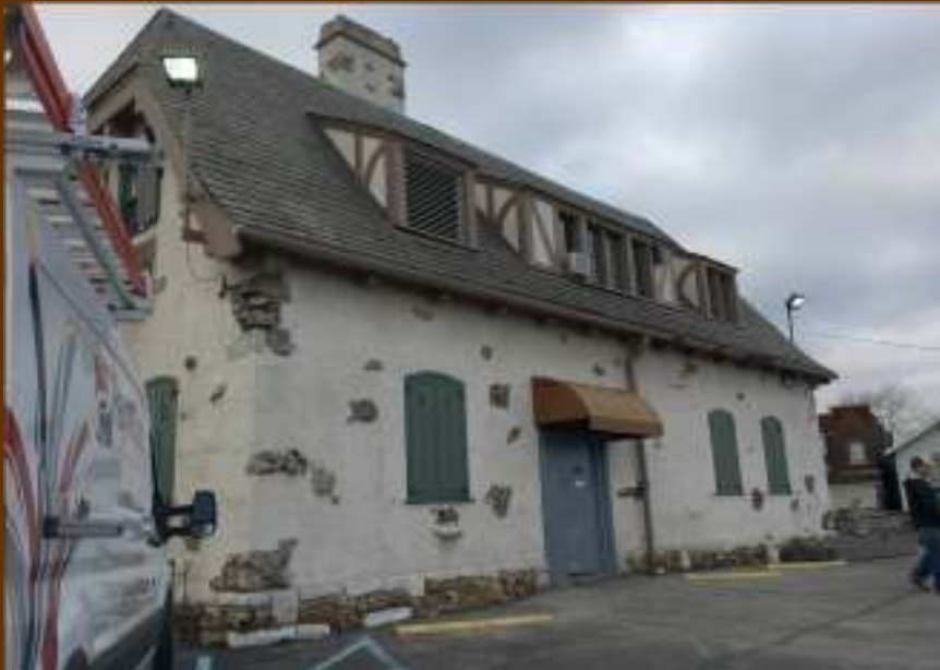
NORTH WALL OF BEVO MILL POINT OF ATTACHMENT
