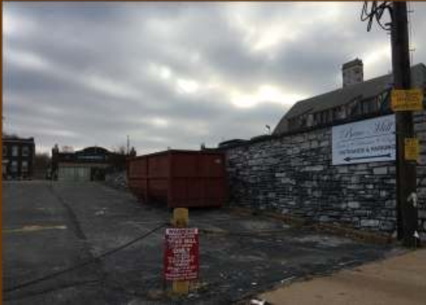
FROM MORGANFORD LOOKING EAST AT RETAINING WALL
