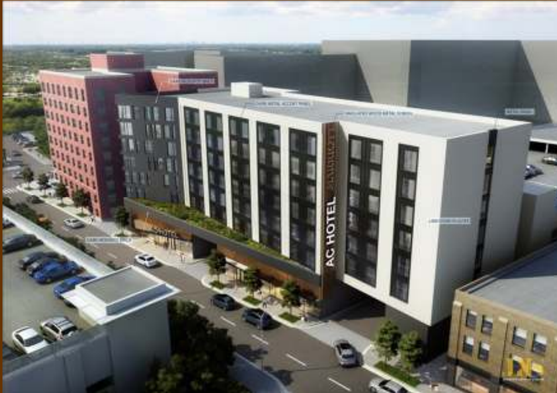
VIEW ALONG YORK LOOKING SOUTHWEST
