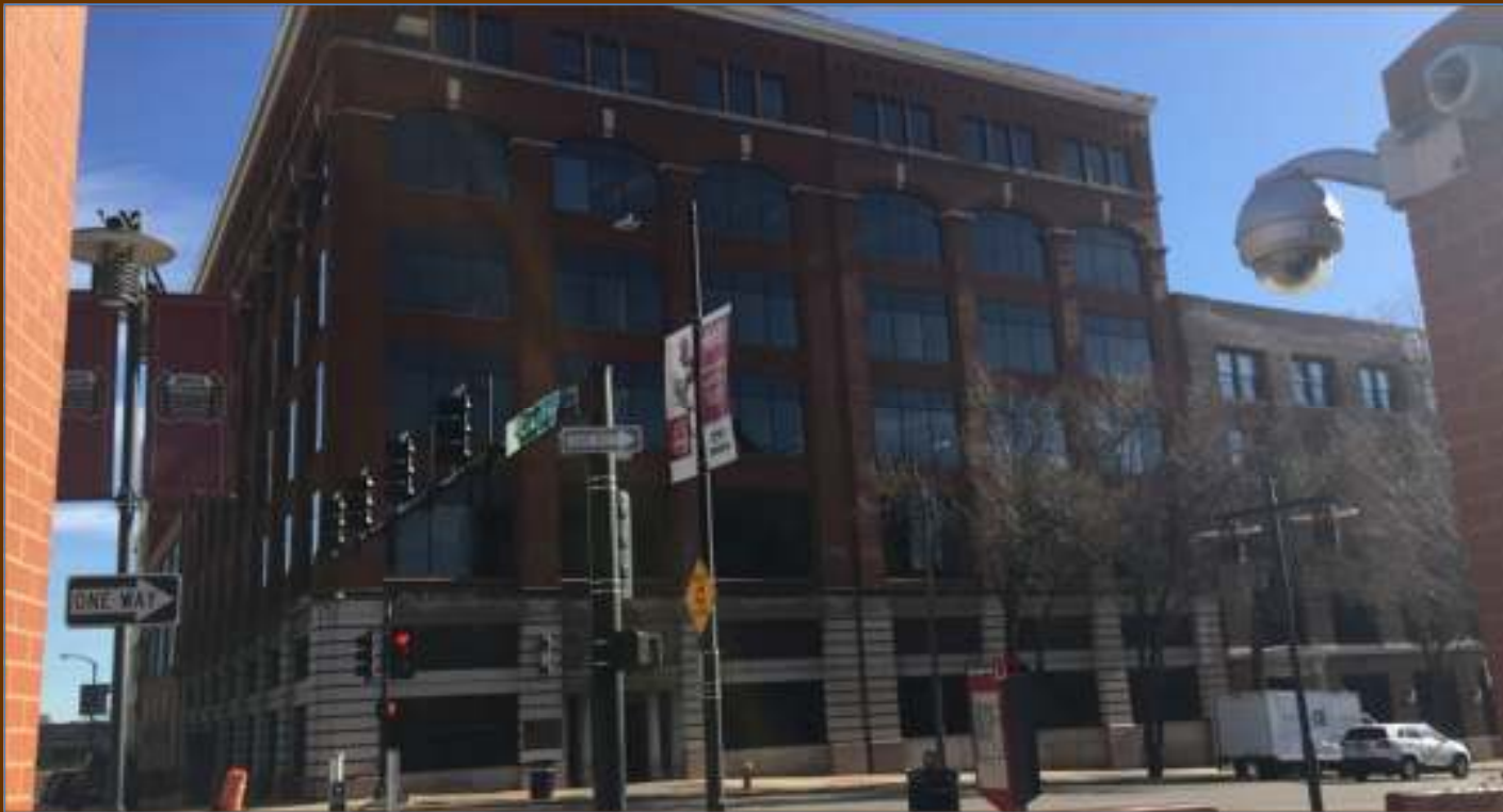
300 SOUTH BROADWAY – PRIMARY FACADE
