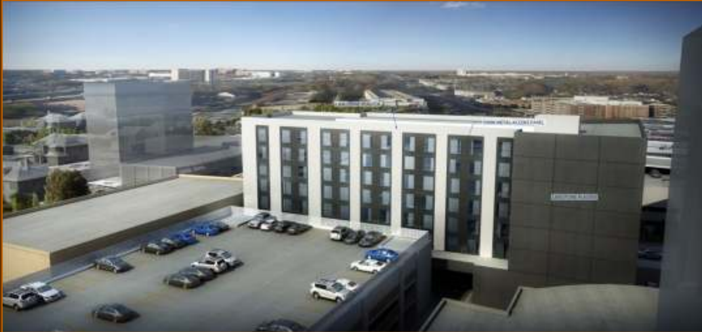
VIEW OF WEST FAÇADE FROM ADJACENT BUILDINGS
