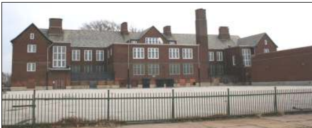
Rear of building showing "E-Plan"
