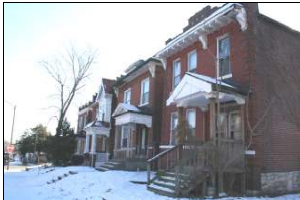
Buildings to east
