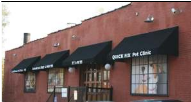
Awning and murals installed without a permit
