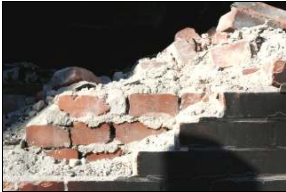
Brick and mortar, side wall
