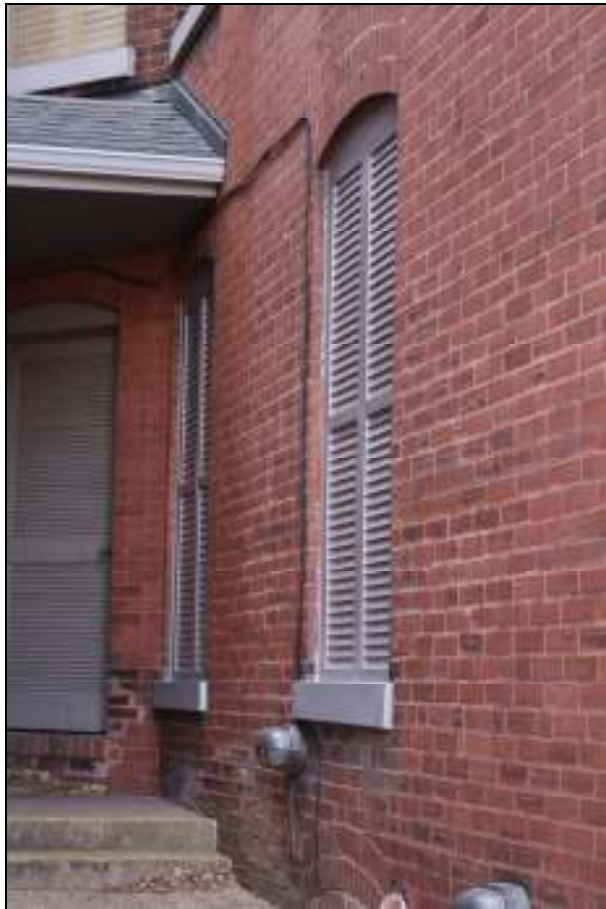
DETAIL OF WINDOWS WRAPPED ON EAST FACADE
