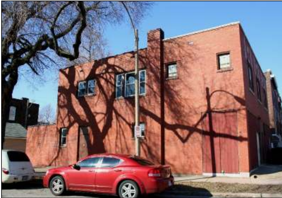
MCNAIR ELEVATION AFTER INSTALLATION
