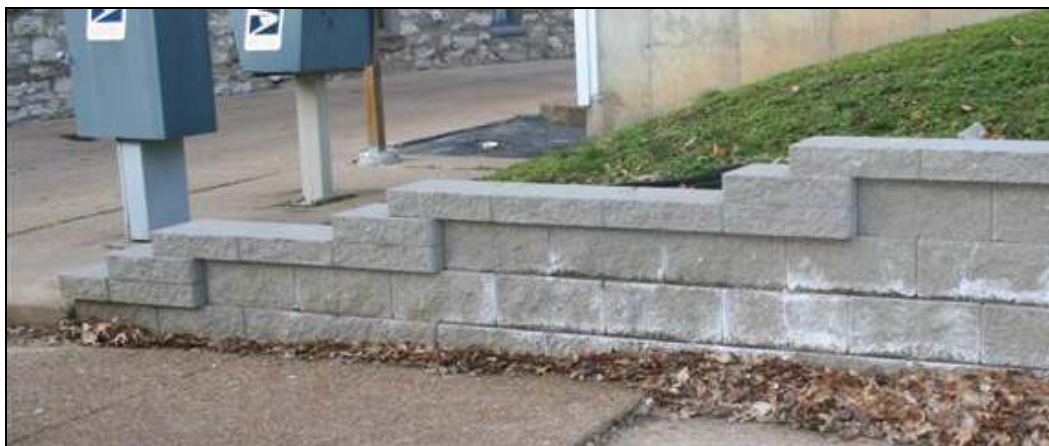
STEPPED END OF INSTALLED RETAINING WALL
