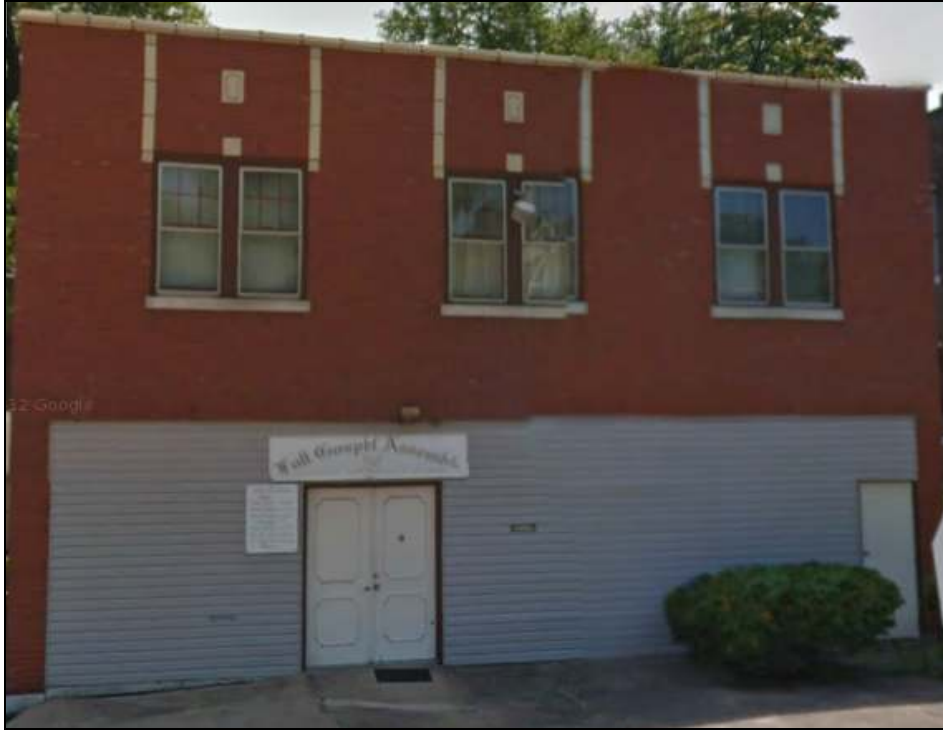
PHOTO OF FRONT ELEVATION BEFORE WINDOW INSTALLATION
