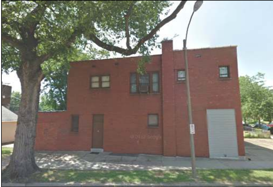
MCNAIR ELEVATION BEFORE WINDOW INSTALLATION
