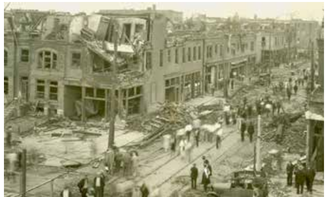
The southern portion of the Vandeventer Neighborhood was extensively damaged by two tornadoes, one in 1927 and another in 1959. These tornadoes damaged homes and businesses displacing people from the area. The photo above shows destruction from the tornado at Sarah and Cook from the 1927 tornado.
