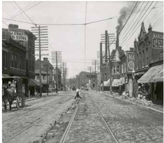
900 Block of Vandeventer with stones, 1921-1923.
