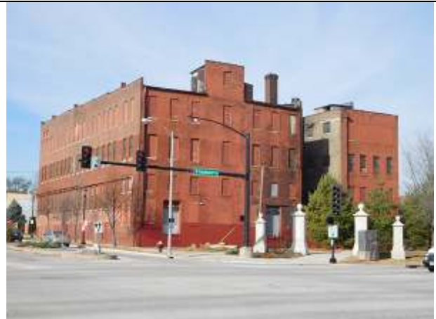
4) Rezoning site Industrial building (Looking southwestward)
