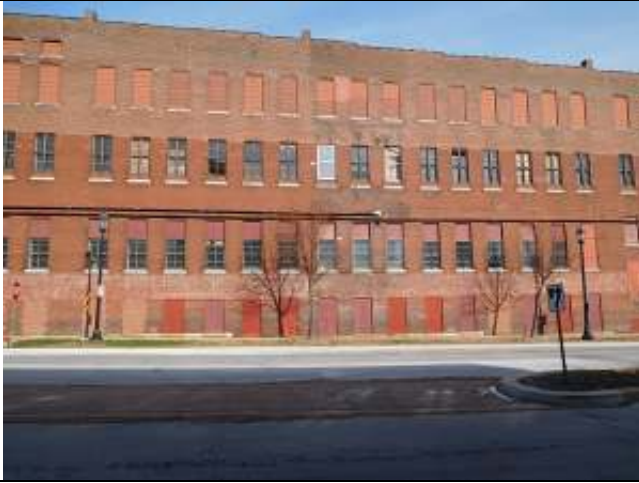
5) Rezoning site Industrial building (Looking northward)
