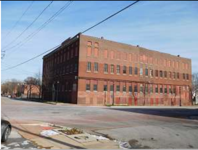
1) Rezoning site Industrial building & parking lot (Looking northeastward)
