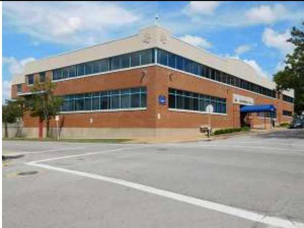
7) Adjacent properties Drummond Hall, 3691 Rutger St. (Looking northeastward)
