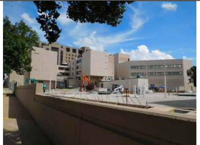
6) Adjacent properties West Pavilion, 3655 Vista Ave. (Looking southeastward)
