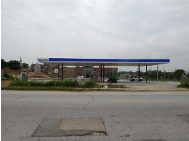
3) Adjacent properties Mobil gas station & Crown Mart convenience store (Looking eastward)
