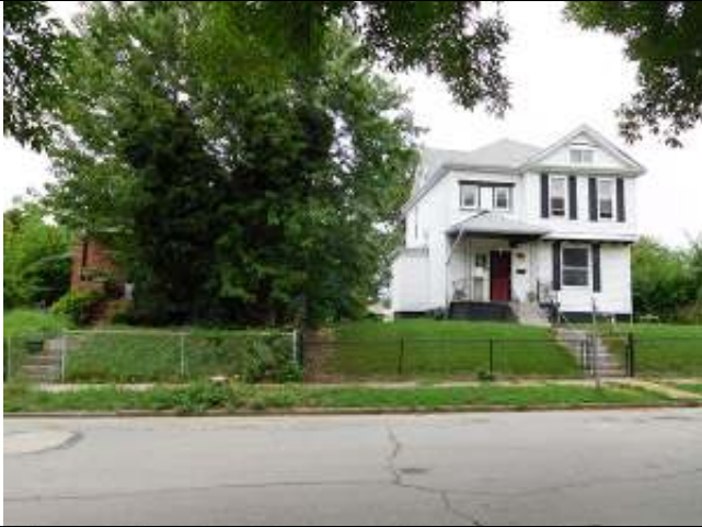
5) Adjacent properties 2 1-family buildings, 4915-19 Geraldine Ave. (Looking westward)
