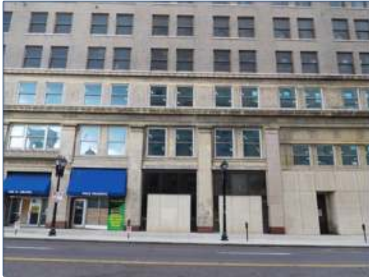
“Blocked-in” storefronts & new windows on 2nd & 3rd floors, 634 N. Grand Blvd.
