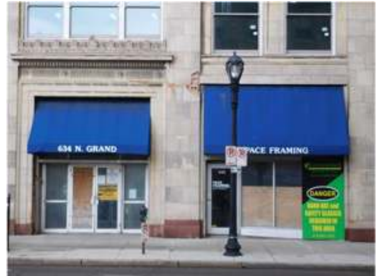
Boarded-up storefronts, 634 N. Grand Blvd.
