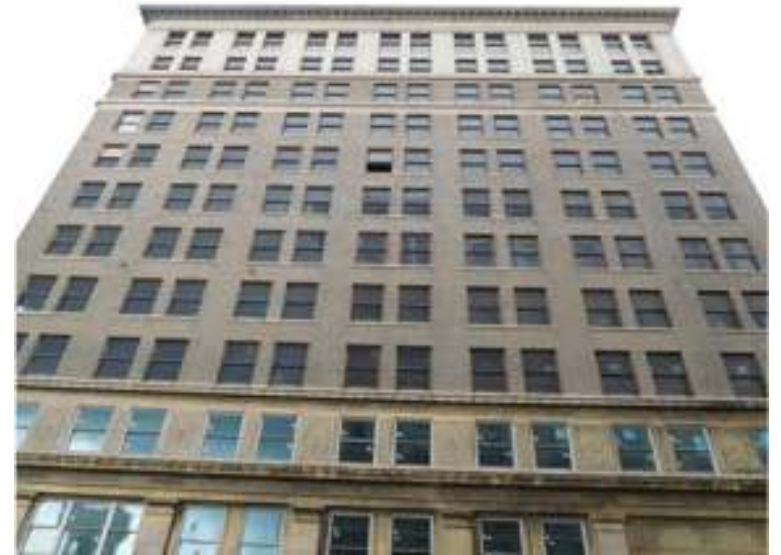
Boarded & open windows, 634 N. Grand Blvd.
