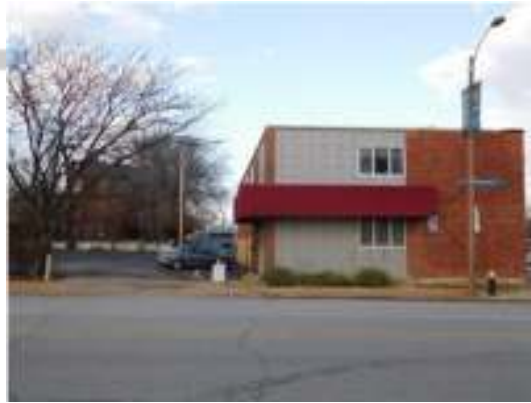
Storage building, 3501 Washington Blvd.
