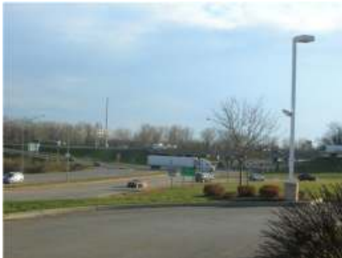
I-270/Riverview Dr. interchange (Looking southward)
