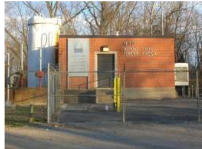
Watkins Creek Pumping Station (Looking eastward)
