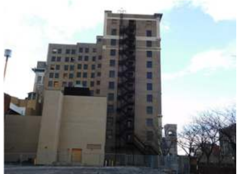
Boarded-up windows & door, 634 N. Grand Blvd.
