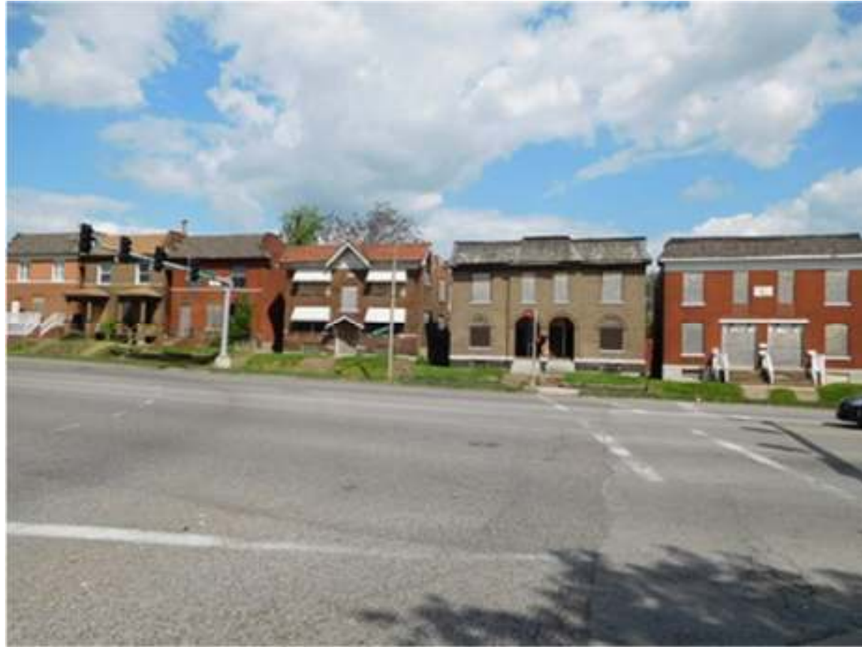
5 vacant & boarded 4-family buildings along 1000 block of S. Kingshighway Blvd.
