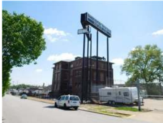
Vacant school building, Sarpy St.
