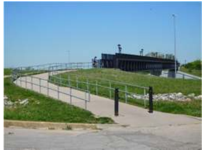
Pedestrian bridge over I-64
