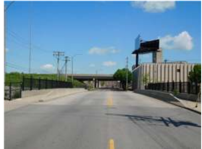
Sarah St. overpass to CORTEX
