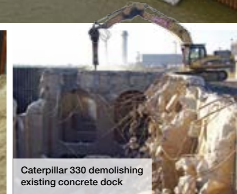
St. Louis Bridge Construction Co
