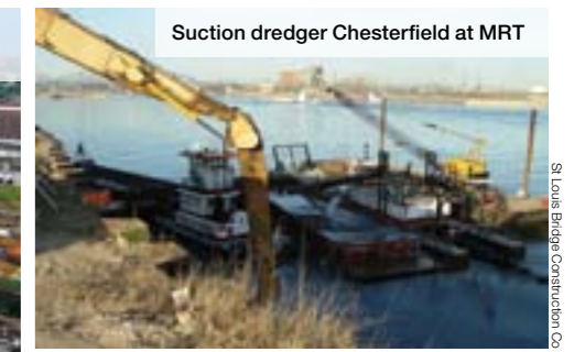
St. Louis Bridge Construction Co
