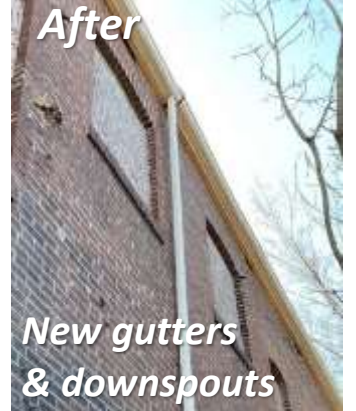
This building features repaired roof with new decking and covering, repaired joists, masonry repairs & tuckpointing, new gutters & downspouts, boarded & secured, cleaned-out & ready for rehab
