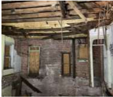
This building features repaired roof with new decking and covering, repaired joists, masonry repairs & tuckpointing, new gutters & downspouts, boarded & secured, cleaned-out & ready for rehab
